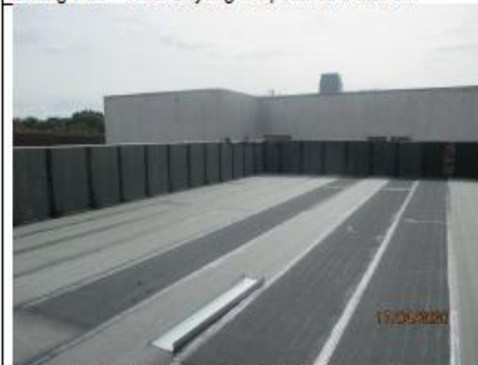
Dining Hall – High Level Roof AVCL In Progress.
