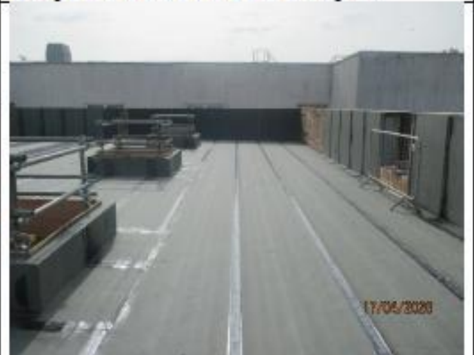
Dining Hall – High Level Roof AVCL In Progress.
