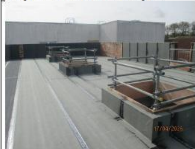
Dining Hall – Roof Sky Light Upstands Installed.
