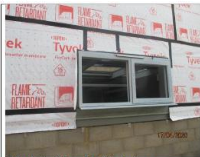
Dining Hall – Window Installation in Progress.
