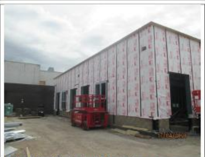
Dining Hall – Window Installation in Progress.
