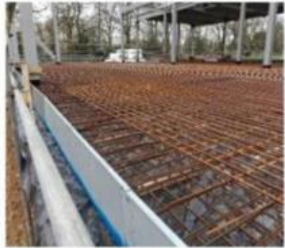
Reinforcement mesh
