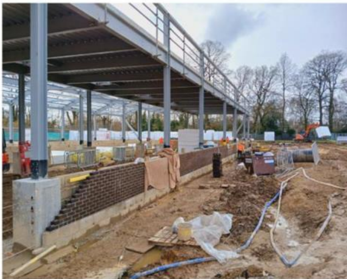
DT Block Slab Preparation Works & Masonry Foundations.
