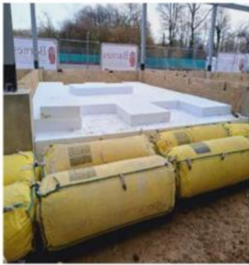
DT Block Slab Preparation Works & Masonry Foundations.
