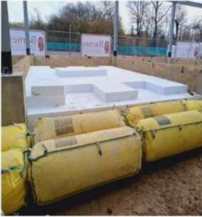
DT Block Slab Preparation Works & Masonry Foundations.
