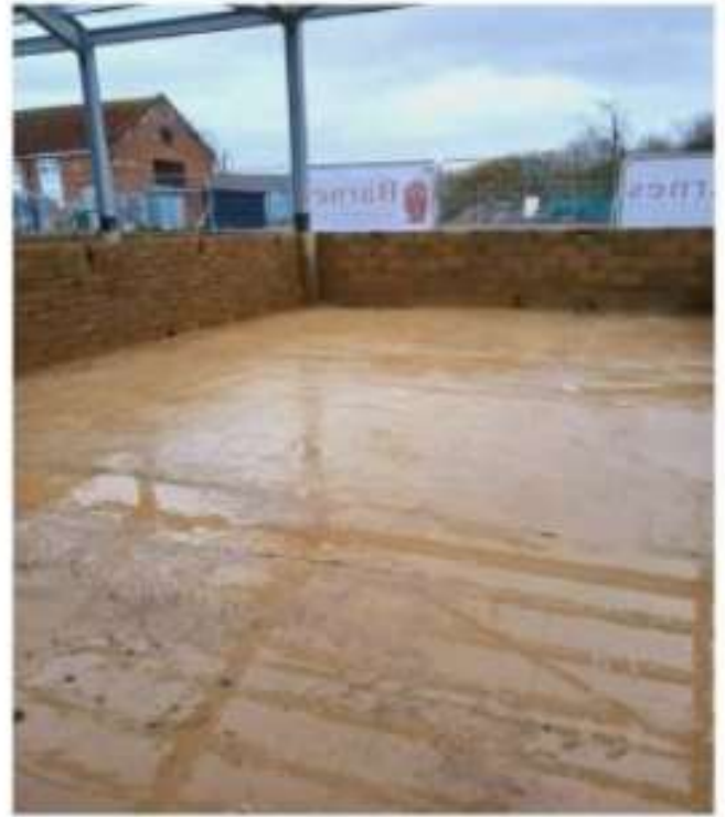
DT Block Slab Preparation Works & Masonry Foundations.
