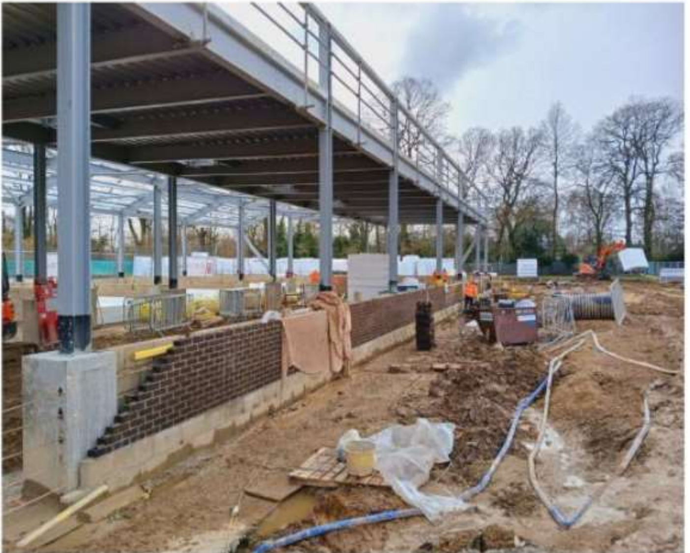
DT Block Slab Preparation Works & Masonry Foundations.
