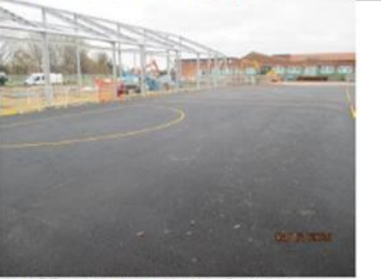
Hard PE – Netball Line Marking Complete.
