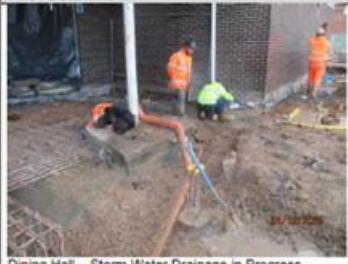
Dining Hall – Storm Water Drainage in Progress.
