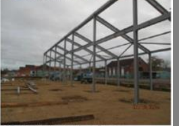
CDT – Steelwork Installation in Progress.
