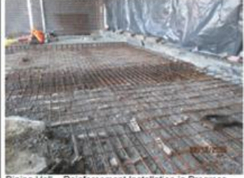
Dining Hall – Reinforcement Installation in Progress.
