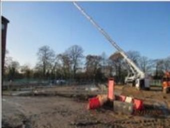
CDT – Steelwork Installation Commenced.
