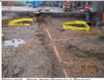
Dining Hall – Storm Water Drainage in Progress.
