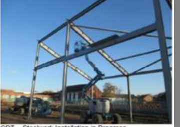
CDT – Steelwork Installation in Progress.
