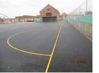
Hard PE – Fence Installation Complete.
