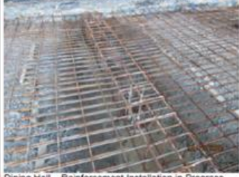
Dining Hall – Reinforcement Installation in Progress.
