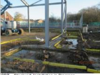
CDT – Steelwork Installation in Progress.
