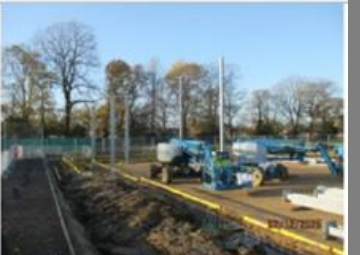
CDT – Steelwork Installation Commenced.
