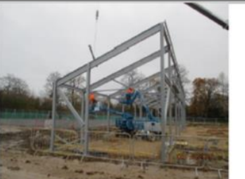
CDT – Steelwork Installation in Progress.
