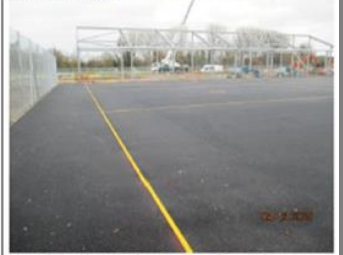
Hard PE – Netball Line Marking Complete.
