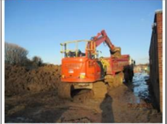
Surplus Soil Removed from Site.
