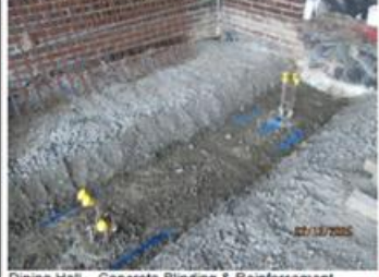
Dining Hall – Concrete Blinding & Reinforcement.
