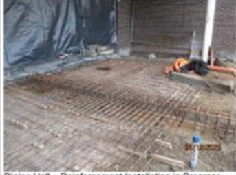
Dining Hall – Reinforcement Installation in Progress.
