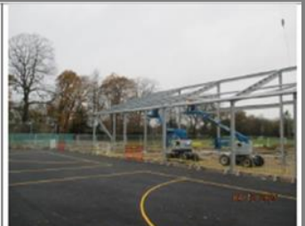
CDT – Steelwork Installation in Progress.
